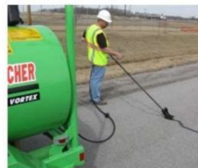
■ Crack Sealing
