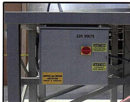
Electrical control panel and agitator timer is enclosed within a single weatherproof NEMA 3R enclosure.
