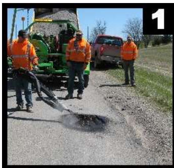
Apply Tack Coat
