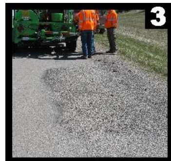
Cover With Dry Aggregate
