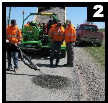
Inject Emulsion Aggregate Mixture
